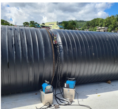
(On-going electrofusion jointing)
